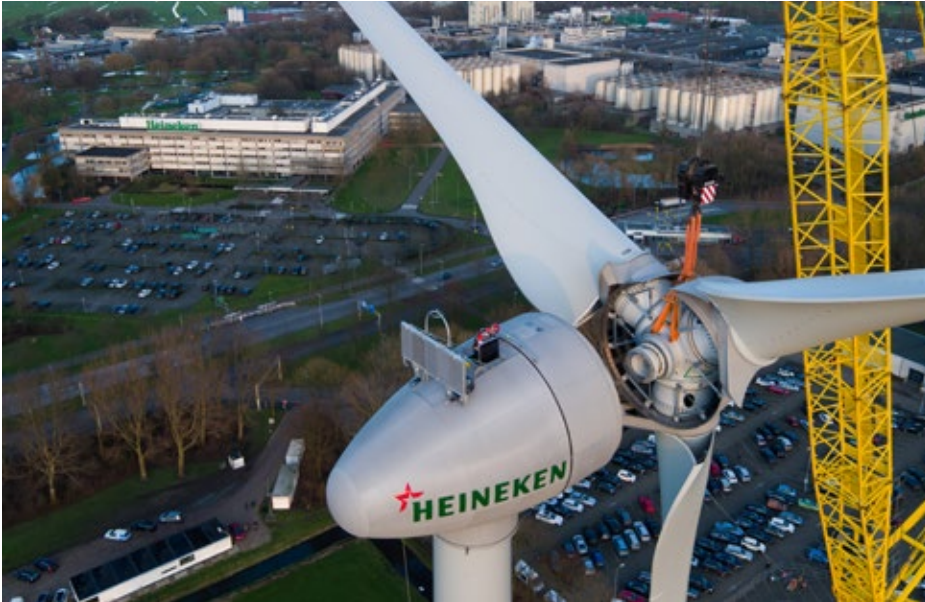
Mounting rotorblades on one of four new wind turbines at our brewery in Zoeterwoude.
